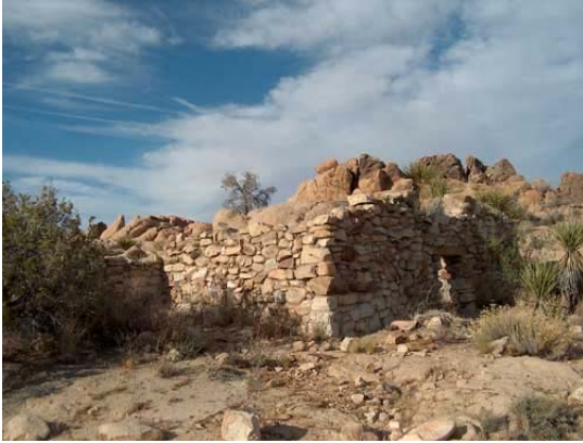
Foundations of rock cabin close to the trailhead
