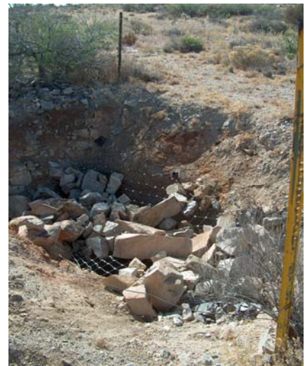
Mineshaft with protective
