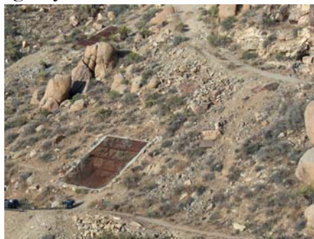
Bat friendly mine shaft covering
